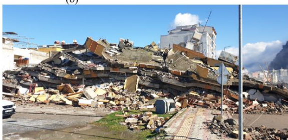
Collapsed buildings having soft and weak stories before and after (map data © 2021 Google): a Sivrice earthquake, b Aegean Sea earthquake, and c M_w=7.7 and M_w=7.6 Kahramanmaraş earthquakes
